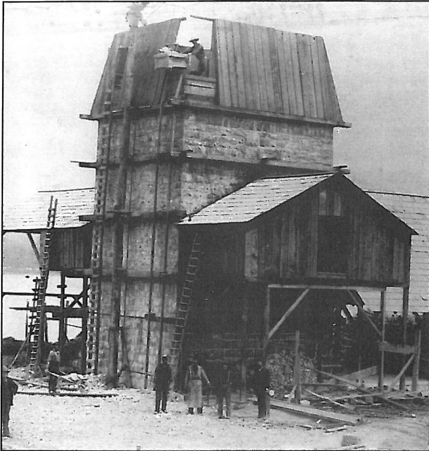
Vancouver, BC: San Juan Lime Company Kiln: many such works were erected in the colonial period to burn limestone and make quicklime (CaO) from which lime mortar was produced. Photo c1888. BCA HP009184
