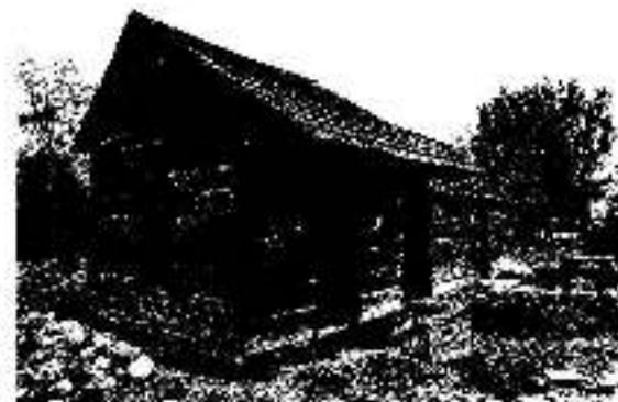
*When the sill logs of the Father Pandey Chapel at the Pimicosis Mission, Kelowna, had rotted, they were removed and replaced with new logs of the same material to consolidate the weakened building.*
