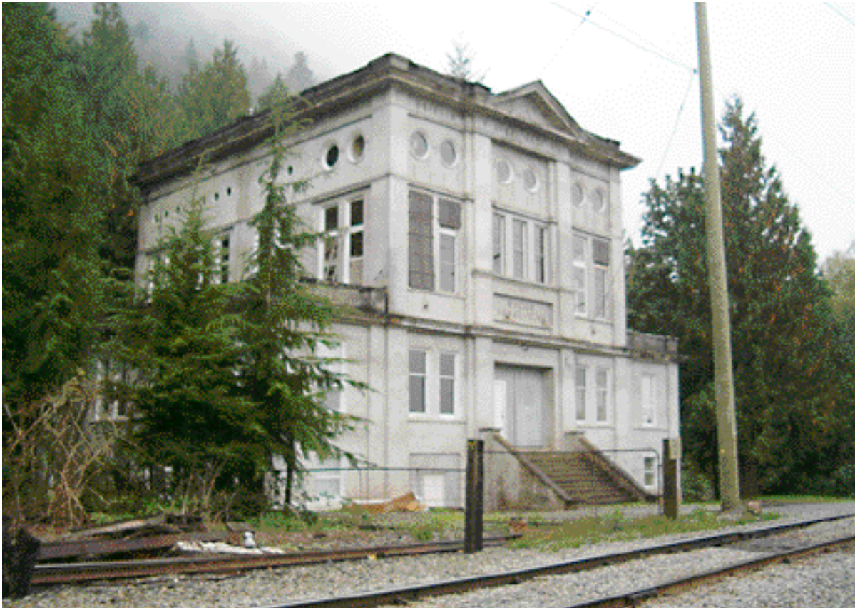
BCER Sumas Substation, Henry B. Watson, Architect, 1909-1910
