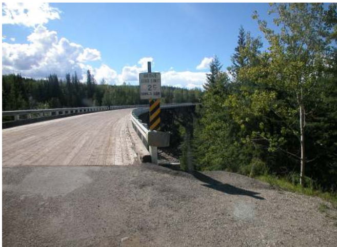
The curved Kiskatinaw Bridge, north of Dawson Creek, is an original Alaska Highway bridge. It has been designated by the Peace River Regional District. (Photo: H. Kalman)
