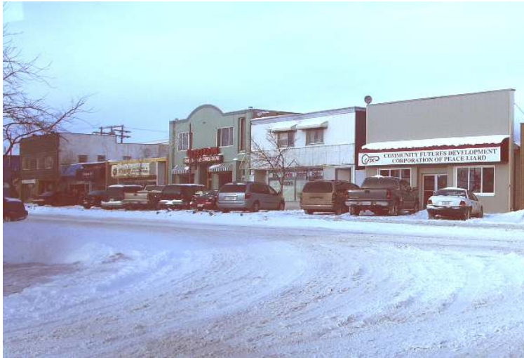
The downtown core retains a number of commercial buildings erected at the time of the arrival of the N.A.R. Most have been altered. This is a view of 102nd Avenue. (Photo: H. Kalman)
