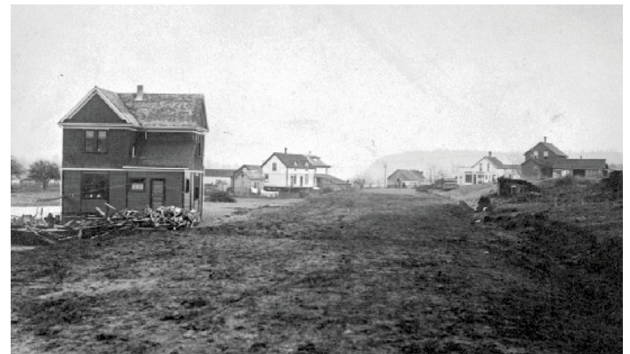
CNR Construction, 1911 (BCA b_07957)
