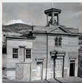
Liberty Fire House, Gold Hill, Nevada. Robert W. Kerrigan, 1937.
