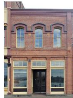
Historic Building – Wharf Street
