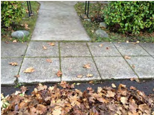
Unique, historic concrete sidewalk with decorative scored pattern.
