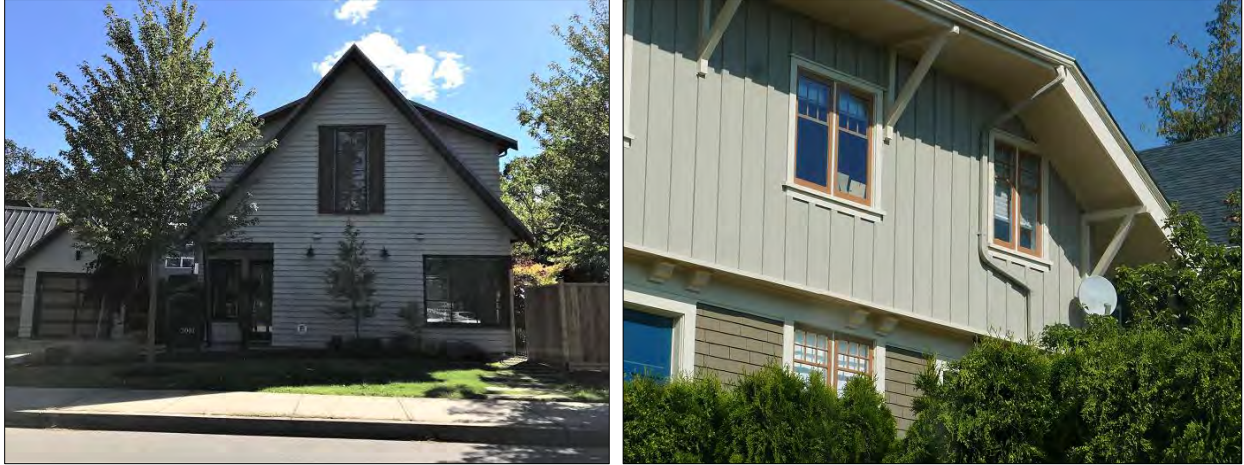
Examples of architectural detailing and forms that are complementary to the historic precedent. The example on the left uses contemporary design and traditional materials to achieve this. The example on the right uses traditional design and traditional materials to achieve this i.e., the detailing in this example is consistent with historic architectural styles in the neighbourhood.
