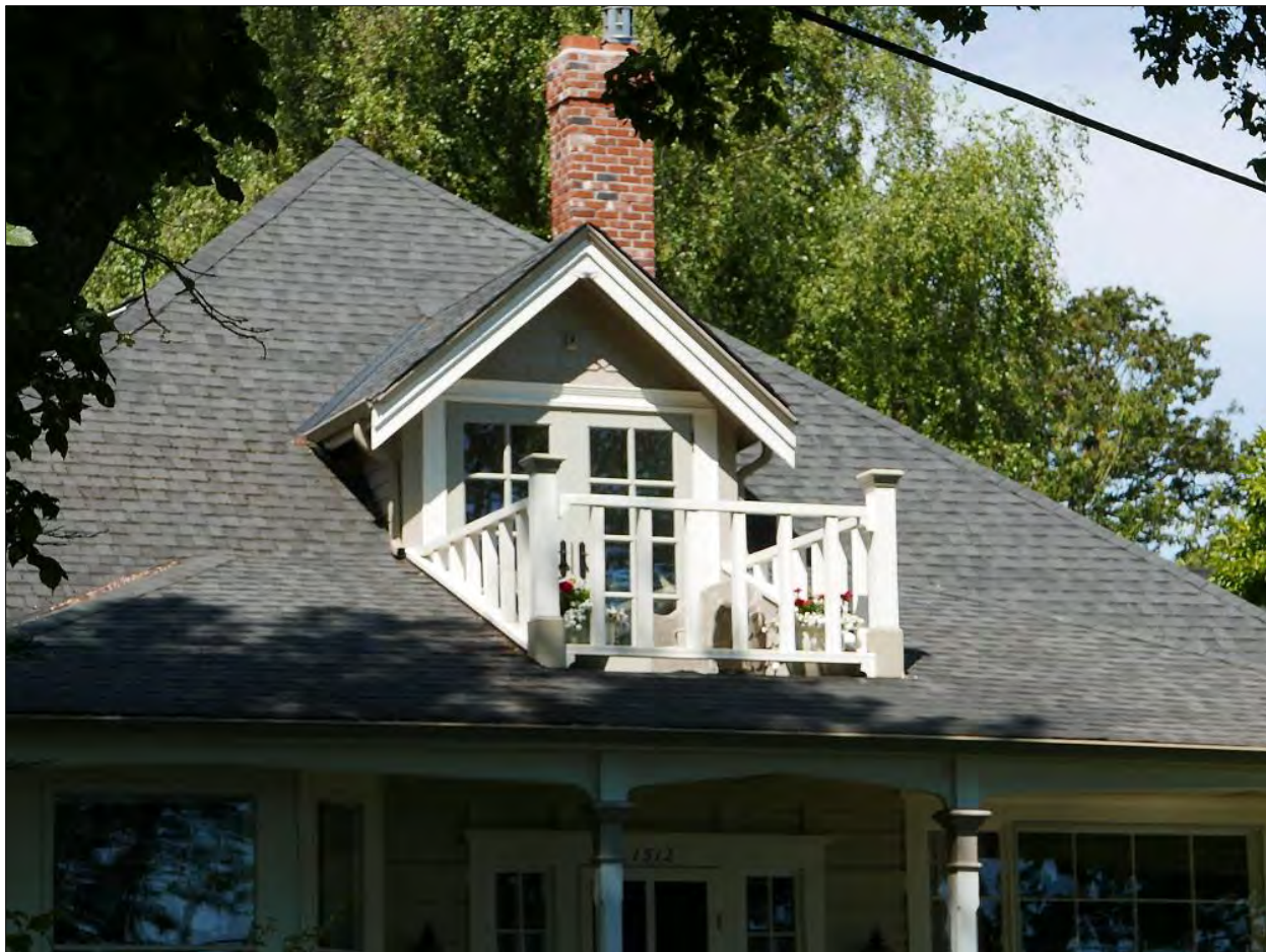
Example of a physically and visually compatible alteration to a protected building in The Prospect. The new dormer uses the same roof pitch as the original roof, and the architectural detailing is consistent with the original period of construction. The materials are also consistent with the original home.
