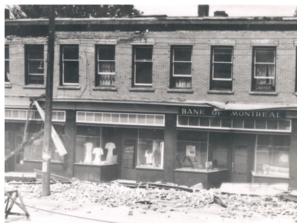
Port Alberni Bank of Montreal, damaged in a magnitude 7.1 earthquake, 1946. Government of Canada https://science.gc.ca/eic/site/063.nsf/eng/97253.html
