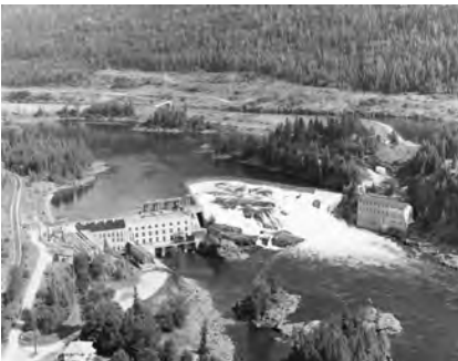
Upper Bonnington dam and powerhouse with Kootenay Canal in background. Photo credit: Nelson Museum, Archives and Gallery
