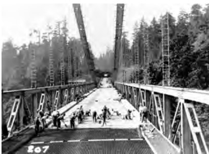
Labourers at work on surfacing the deck of the Lions Gate Bridge, 1938. Photo credit: NVMA, 5294
