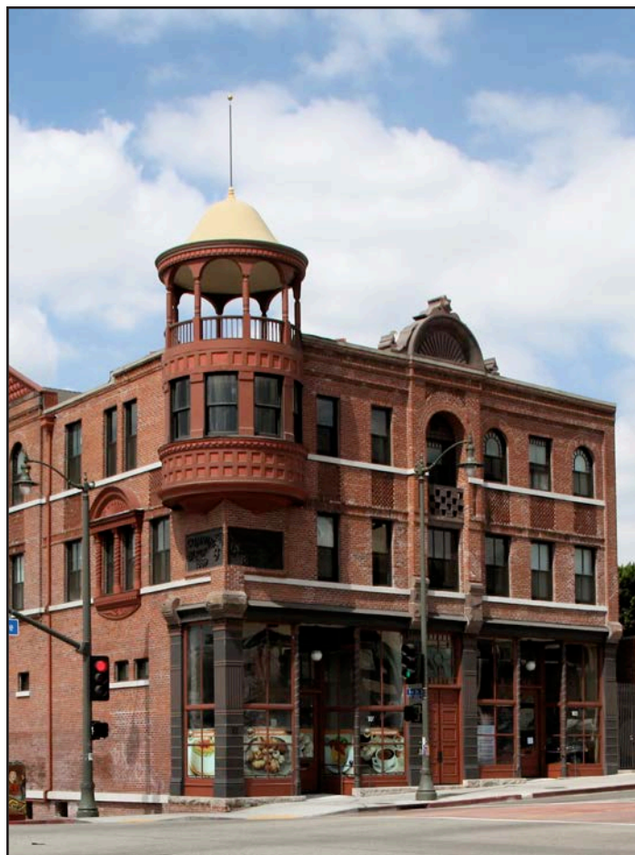
Fig. 5.4: The Boyle Hotel, in East Los Angeles, is an example historic unreinforced masonry (URM) building that received funding from the Federal Historic Preservation Tax Incentive Program for rehabilitation to allow for continued use. (Source: Bruce Bohner)
