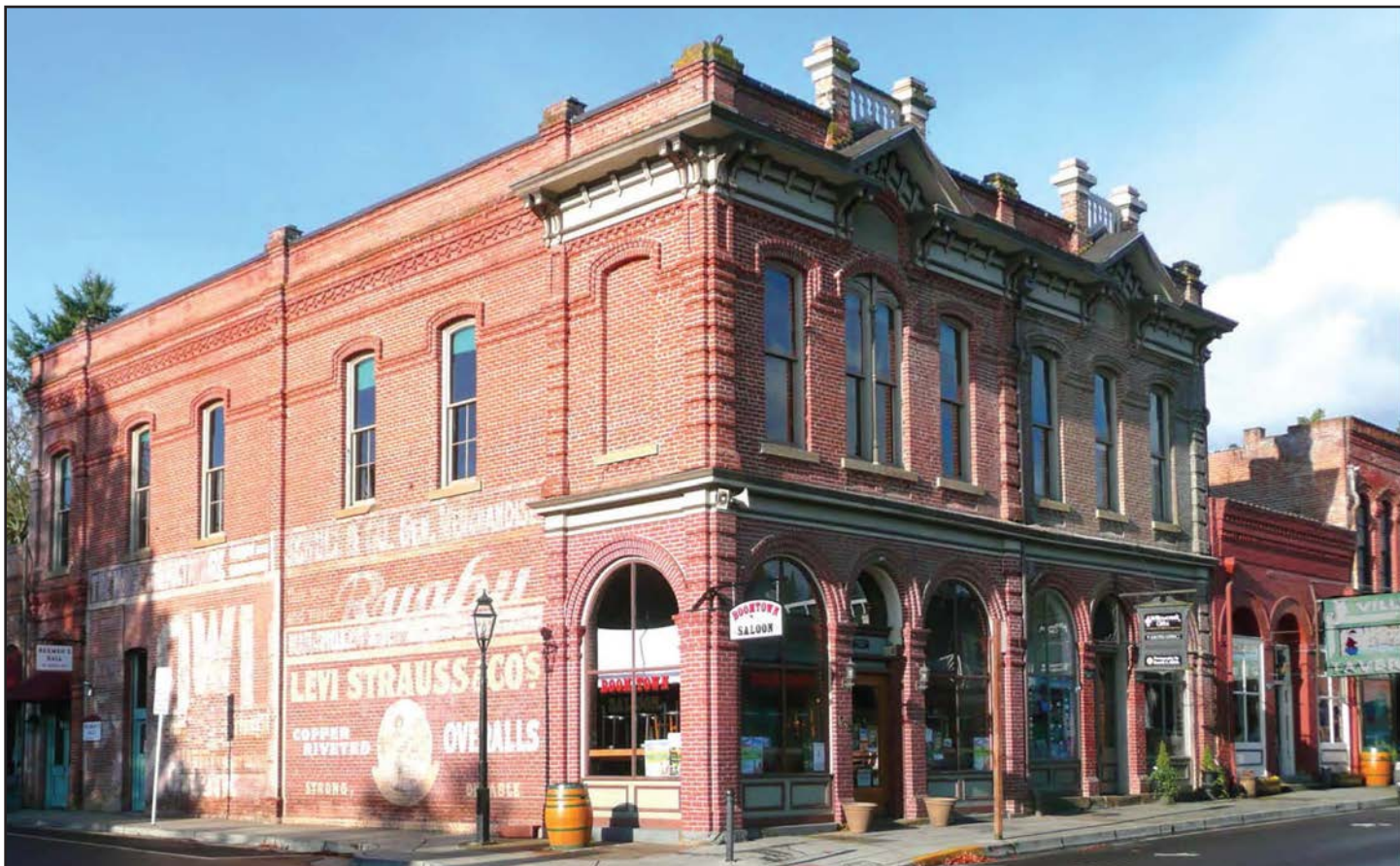
Fig. 5.9: Redman Hall from Jacksonville, Oregon, illustrating one of its seismic at-risk URM buildings. (Source: Restore Oregon)
