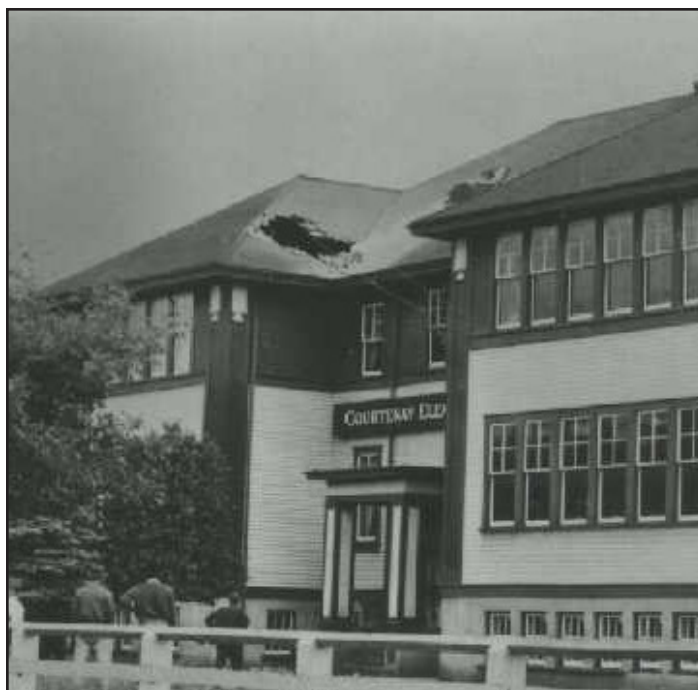
Fig. 2.5: Courtenay School earthquake damage, exterior, 1946. (Source: Courtenay & District Museum (CDM))
