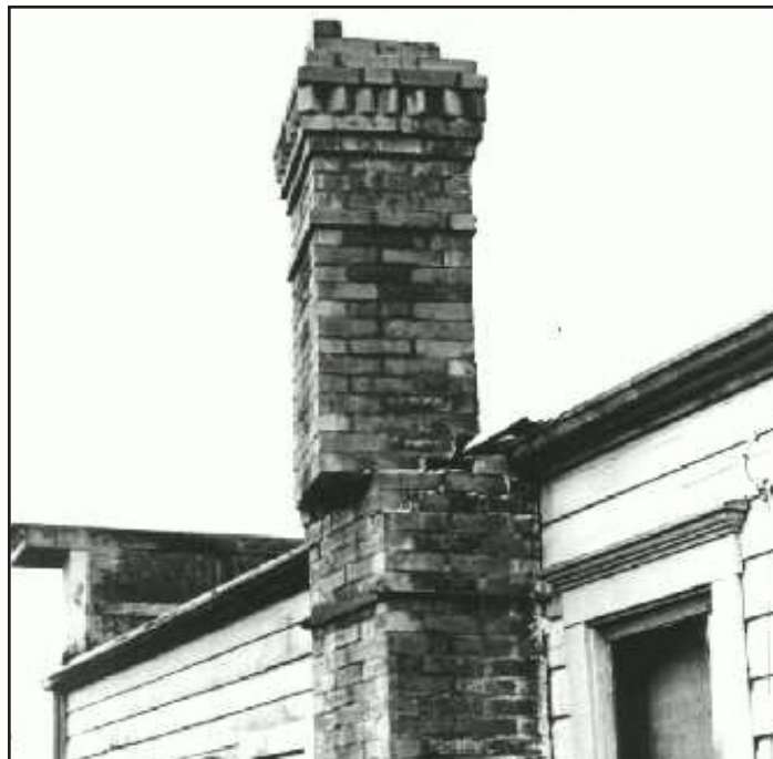
Fig. 2.7: Port Alberni Chimney Damage, 1946, over 70 km away from the earthquake's epicenter. (Source: CDM)
