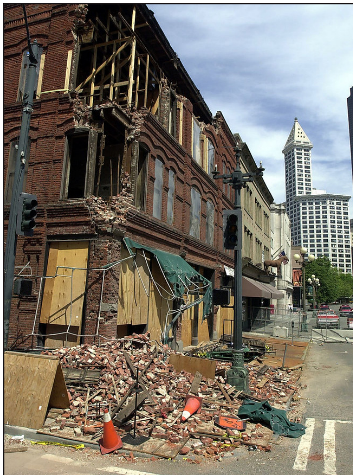
Fig. 5.13: Damage in Seattle from the 2001 Nisqually Earthquake. (Source: Northwest Progressive Institute)
