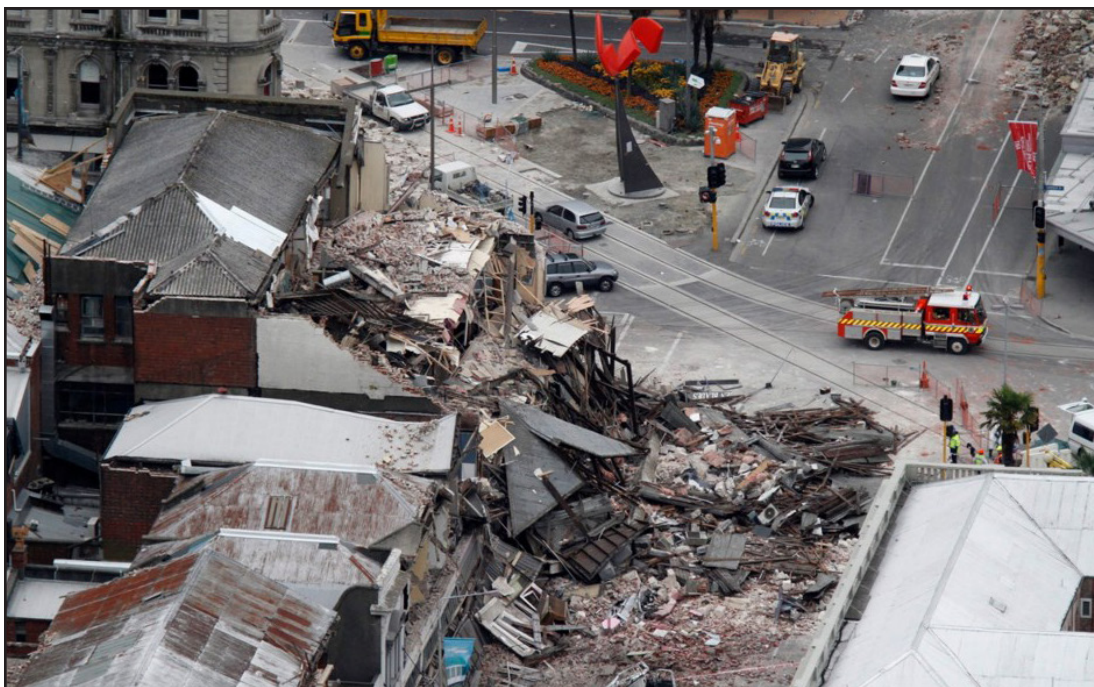
Fig. 5.28: Earthquake damage experienced in Christchurch's Central Business District, at the intersection of Lichfield, Manchester and High Streets in Christchurch, 2011. (Source: Mark Mitchell)
