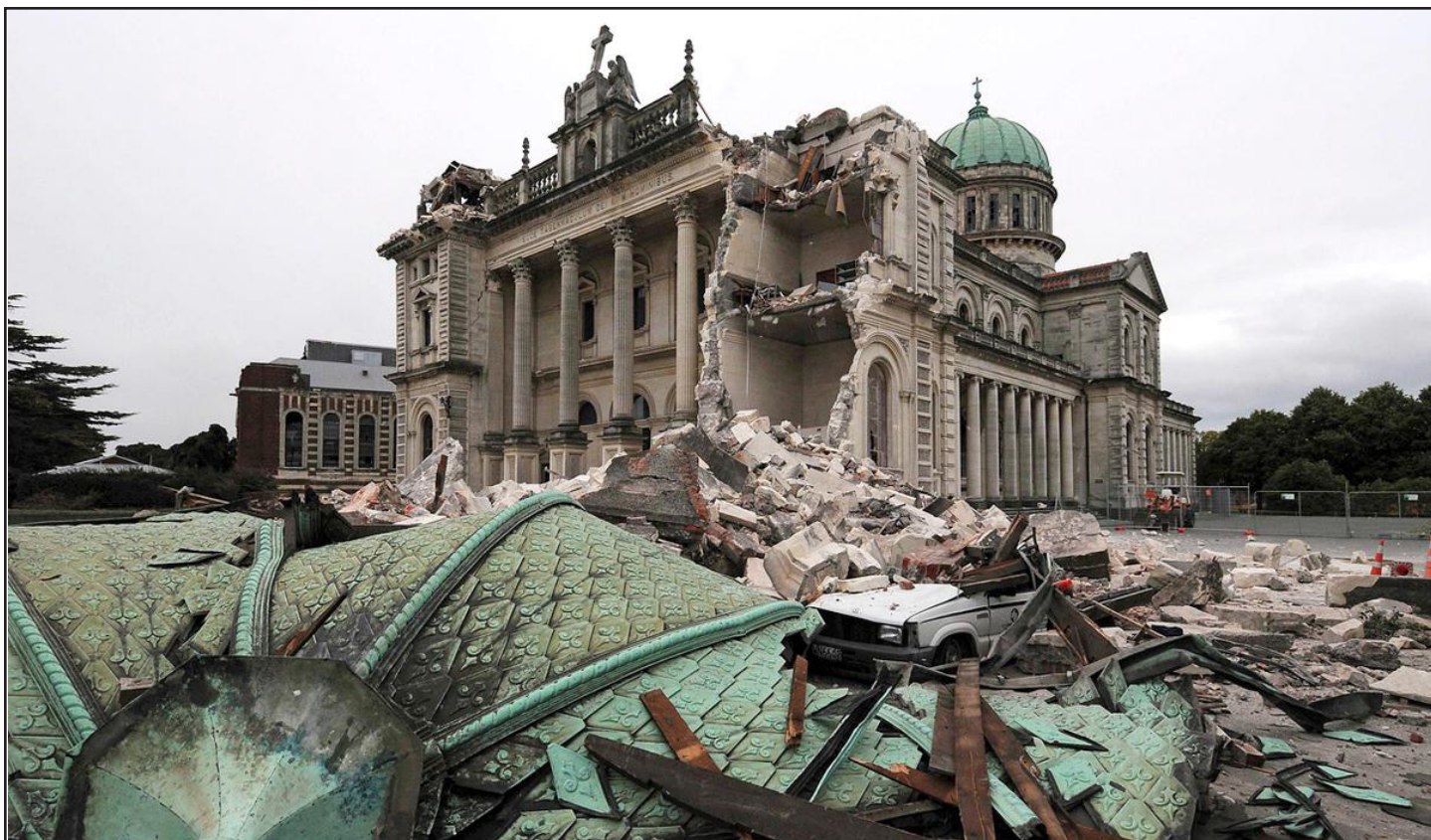
Fig. 5.27: Cathedral of the Blessed Sacrament partially collapsed in the February 2011 Christchurch earthquake. After eight years of debate and the site left in disarray, it was decided in 2019 to demolish the remaining sections of the Category I heritage-listed structure from 1905. (Source: New Zealand Press Association, David Wethey)
