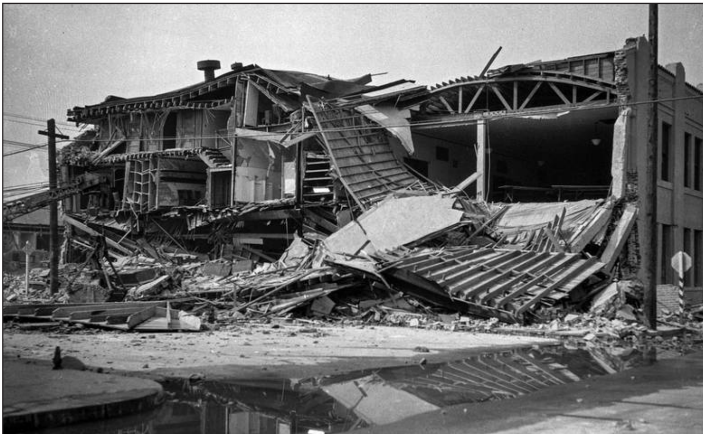
Fig. 2.12: Example earthquake damage, showing a partially collapsed Masonic Temple from the 1933 Longbeach earthquake in California. (Source: The LA Times Archive)
