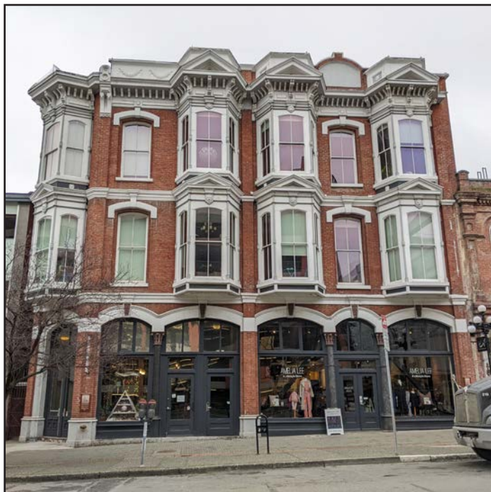
Figs. 3.1a & b: Example late 19th and early 20th century brick buildings in British Columbia. The bottom building has had some retrofit work done, as visible in the store window with the black diagonal bracing. (Sources: Katie Cummer)
