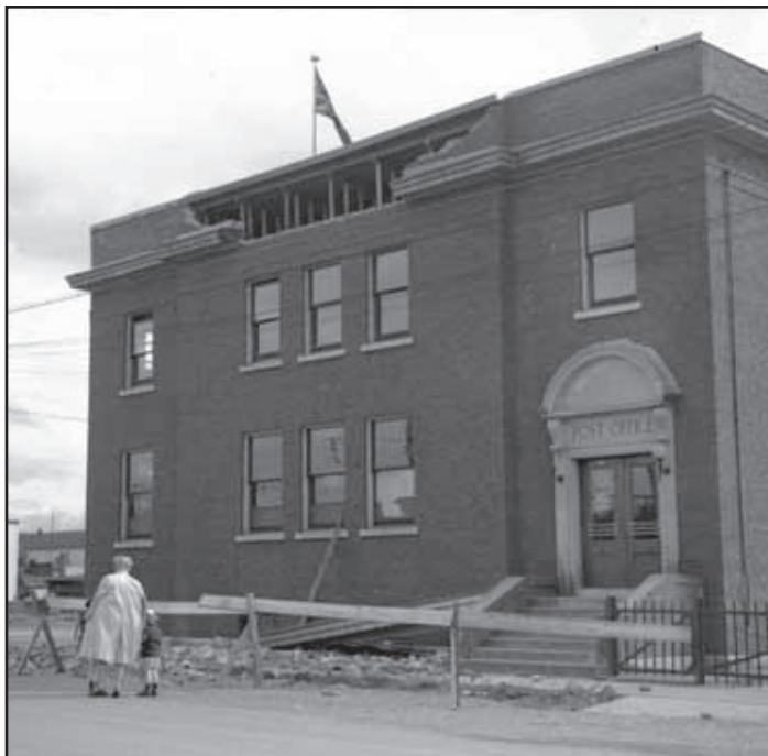
Fig. 2.3: Courtenay Post Office earthquake damage, 1946. (Source: Vancouver Public Library, 41749)
